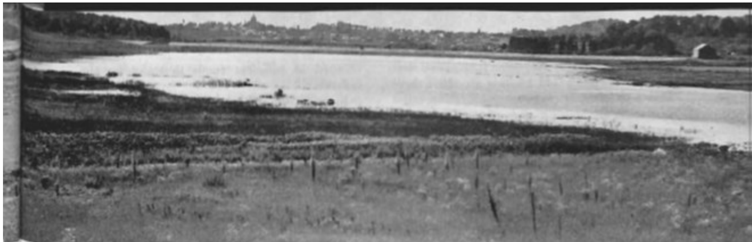
PRESENT VIEW looking toward the dam breast. IN THE background is Somerset Borough.
